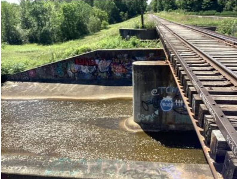
Downstream of spillway
