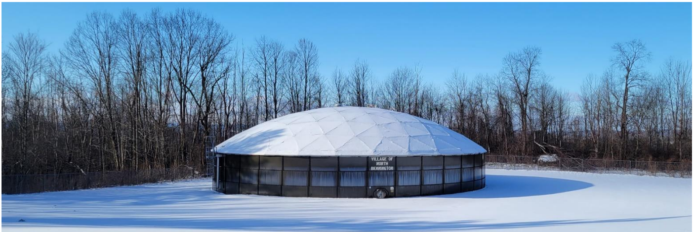
North Bennington Water Storage Tank.
