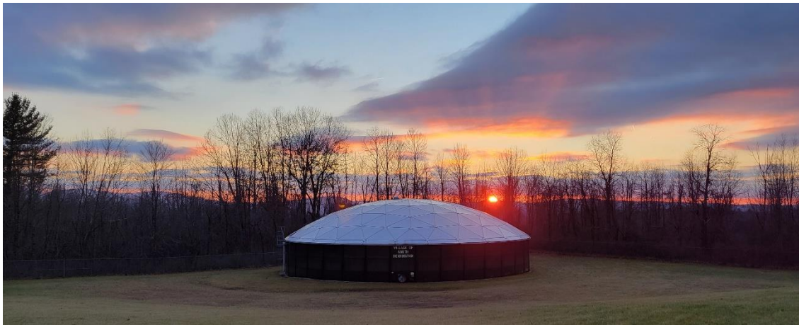
North Bennington Water Storage Tank.
