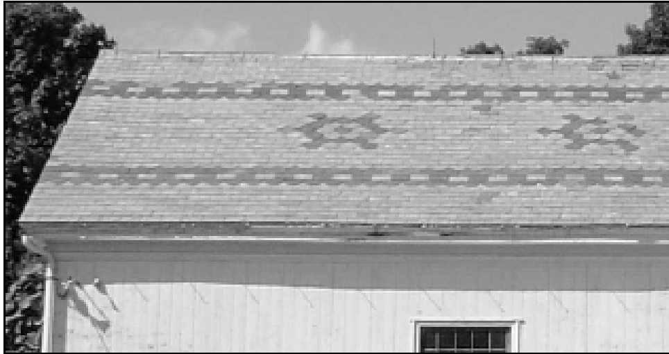
Figure 27. This creative pattern on a slate roof is an excellent way to enliven the design and break up the expanse of the roof.
