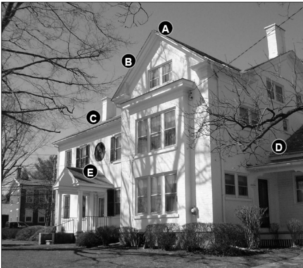
Fig. 9: Roof Design. The many different roof elements seen here help to break up and reduce the scale of an otherwise large house.
