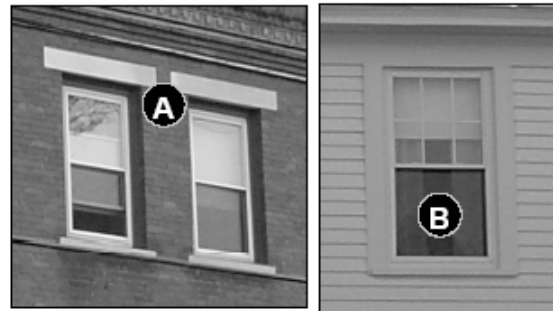
Fig. 25: Examples of proper window treatment. The brick building expresses the structural lintel above the window. Both photos show the storm window is painted and recessed within the window opening.
