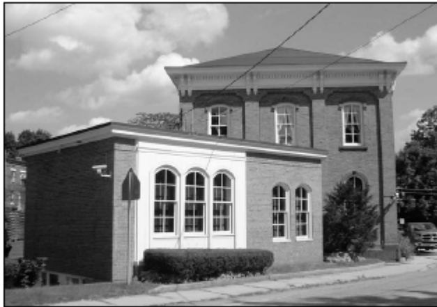
Fig. 21: Although the windows on the new addition don't exactly match the original windows on this bank, they are generally the same in style and proportion, helping to tie the design together.
