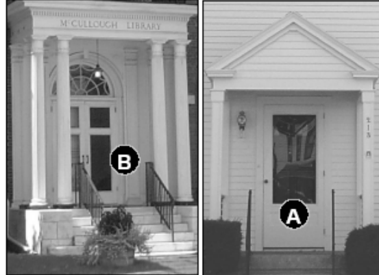
Fig. 23: Examples of proper storm doors. These wood doors are mounted flush with the door trim, and do not contain any unnecessary detail which would detract from the original door design.
