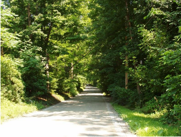
The narrow road profile, gravel surface, and mature trees that arch over the roadway make Park Street a particularly scenic road and an important community asset.
