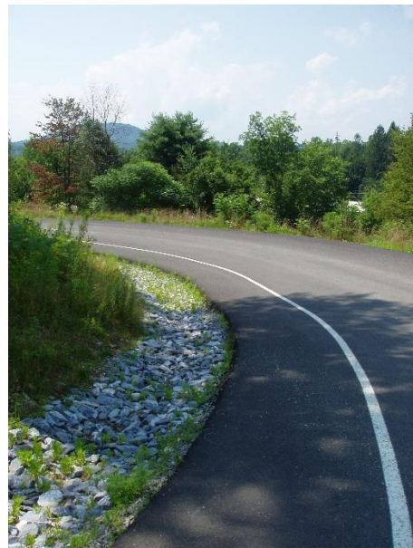
Private roadways must be designed to meet Village standards, providing for features such as good pavement, markings for bicycle and pedestrian travel, and proper drainage ditches.
